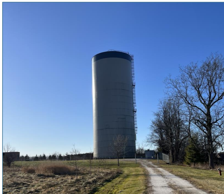
Photo of Existing Tank
